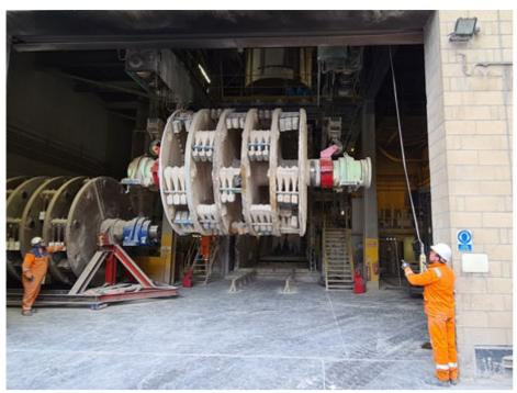
Hoist and Winch helped a cement industry customer replace a large rotor used in its production process.
